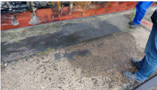
picture 1: vessel made oil spill on berth
