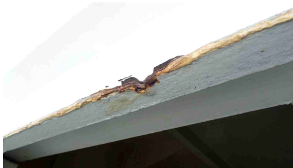
picture 22: tight closing not possible with this frame
