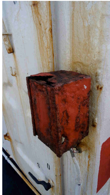
picture 41-43: fluent passage from poor external structure, rusted cover and poor condition of switch
