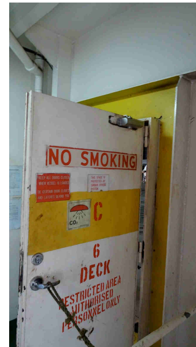
picture 55-57: fire doors were found damaged, bent, kept open by ropes, not more self closing or not tight closing
