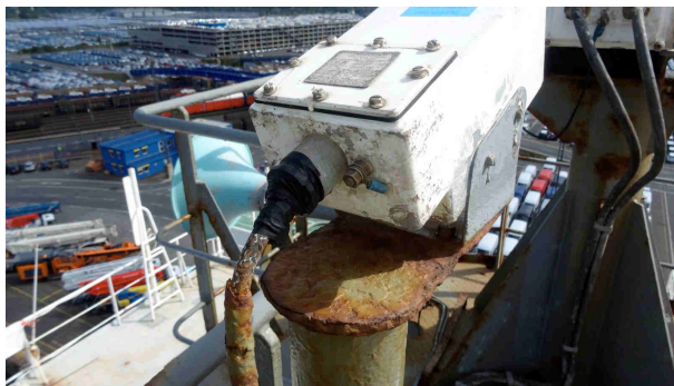
picture 38: destroyed insulations were...
