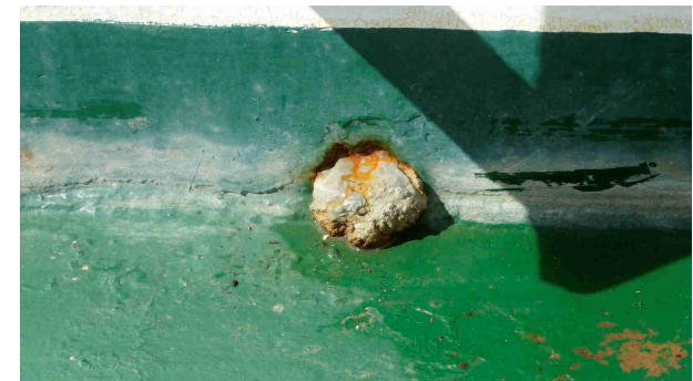
picture 53: ...some of them filled by concrete
